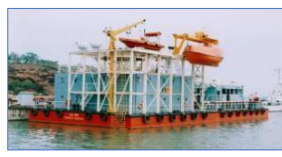
Survival at Sea Training Facility FPR for ONGC
