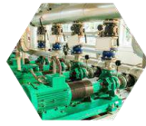
Welding, Pumps & Piping
