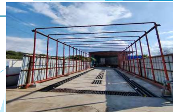
Shower Testing Area
