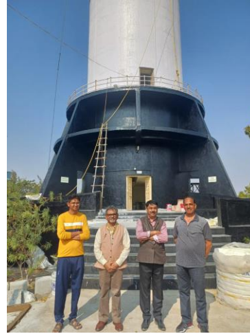
Mandavi Lighthouse Renovation on 12.02.2026
