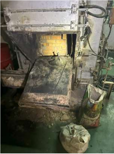
Non operational incinerator
