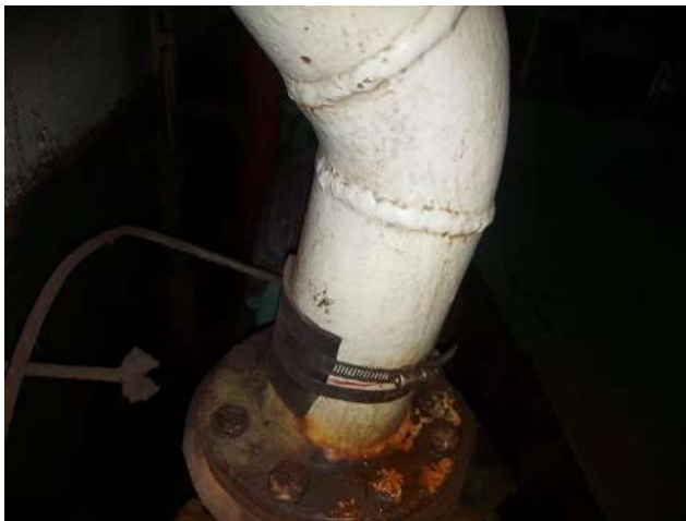
Temporary repairs on S/W Pipeline
