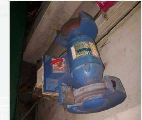
No protection. Guard
