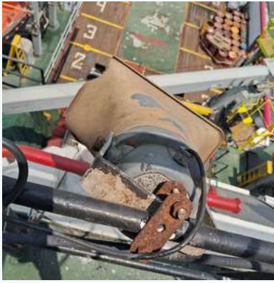
Damaged Public Address Systems
