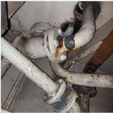
AC sw cooling overboard line repaired with devcon
