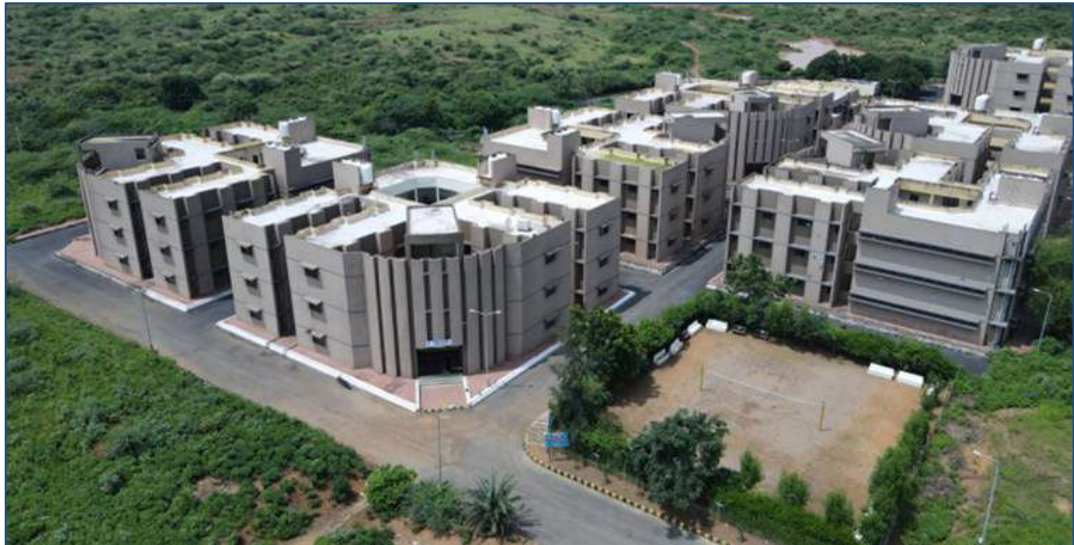
Figure 2-16: Accommodation complex for workers
