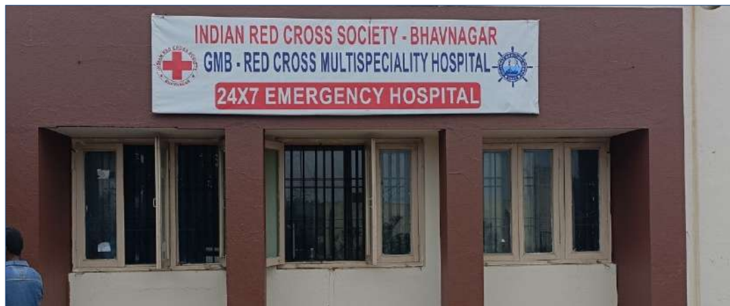
Figure 2-15: Multi specialty hospital at Alang
